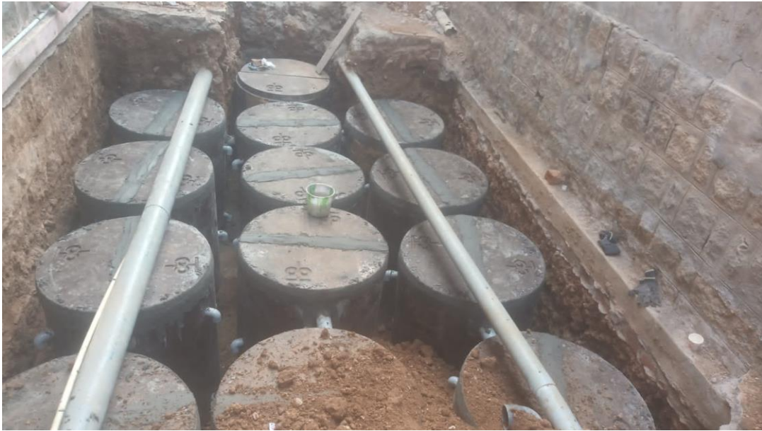
Bio water Treatment Process inside the campus
